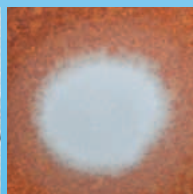
Rusted sheet iron
